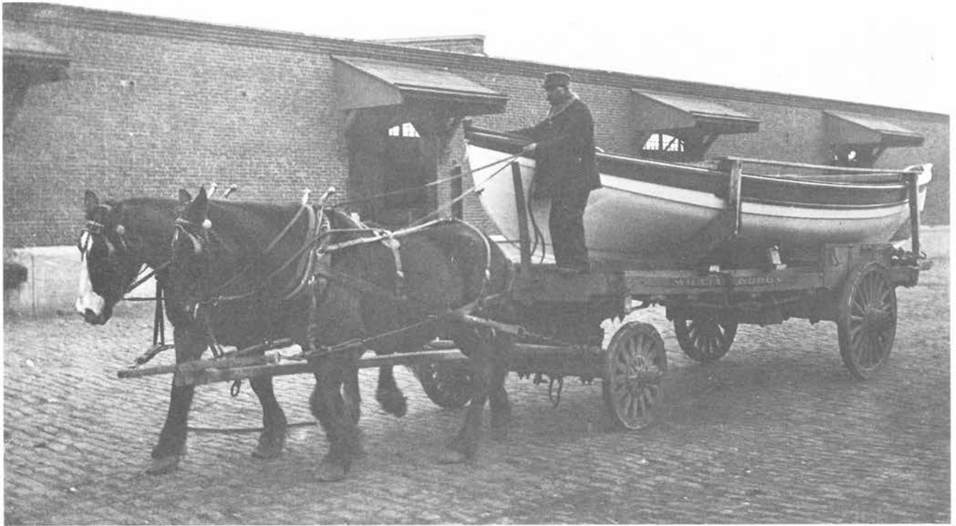
Figure 4-28. Boat shops located in New Bedford could hire a local teamster to deliver their boats if it was not convenient to put them overboard at the shop and deliver them by water. Boats were frequently stored in open fields or empty lots in many parts of the city, necessitating their transport by wagon. From a negative by Albert Cook Church. Old Dartmouth Historical Society
