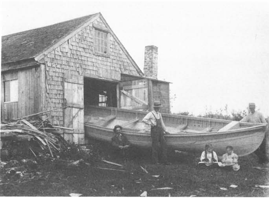
Figure 4-25. The Leonard boat shop, Acushnet, Massachusetts, circa 1900. The finished boat is being eased out of the shop for transport to New Bedford on a wagon. The outbuilding to the right of the shop entrance houses the oven and kettle for the steam box. Old Dartmouth Historical Society
