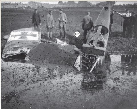
The crash and recovery of DFW C.V (LVG) 'white 4' from Schusta 26 allows us to see several interesting details. Note the style of the exhaust which is almost exclusively found on LVG built DFW C.V, the small support brackets from the cabane to the radiator and the square white fields behind the wing and fuselage eisernkreuz. These white fields were eliminated in a directive sent in October 1916 which would indicate that this aircraft is from a production order placed that month with LVG for 50 DFW C.V (numbers 7650/16 to 7699/16).
