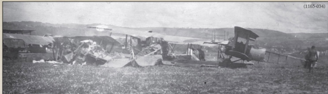
No longer required by the USAS following the Armistice these 186th Aero Sqn Salmson 2-A2, similarly stripped of their colourful markings for souvenirs, await destruction.
