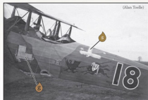
Salmson 2-A2 '18' showing some repaired 'battle damage' above the unit insignia and patched fuselage fabric covering a previous installation of the external generator partially hidden by Phil Henderson in this photo.
